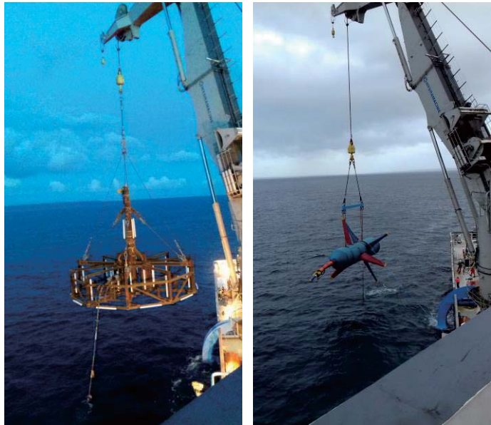
Fig. 1 Example of a pre-commercial tidal turbine installation.
